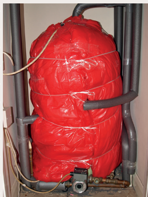
Hot water cylinder in airing cupboard (wrapped in fibre glass insulation jacket)
