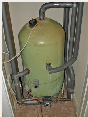
Hot water cylinder in airing cupboard (without insulation jacket)
