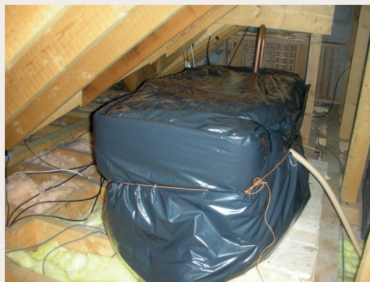
Cold water storage tanks in loft space
