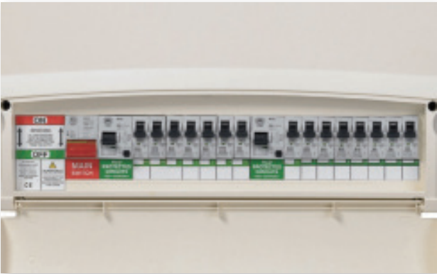
Fully RCD protected, all trip switches green No upgrade work needed.
