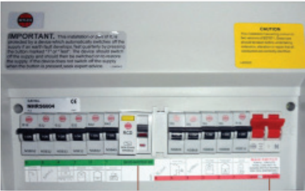
Fully RCD protected, all trip switches green No upgrade work needed.
